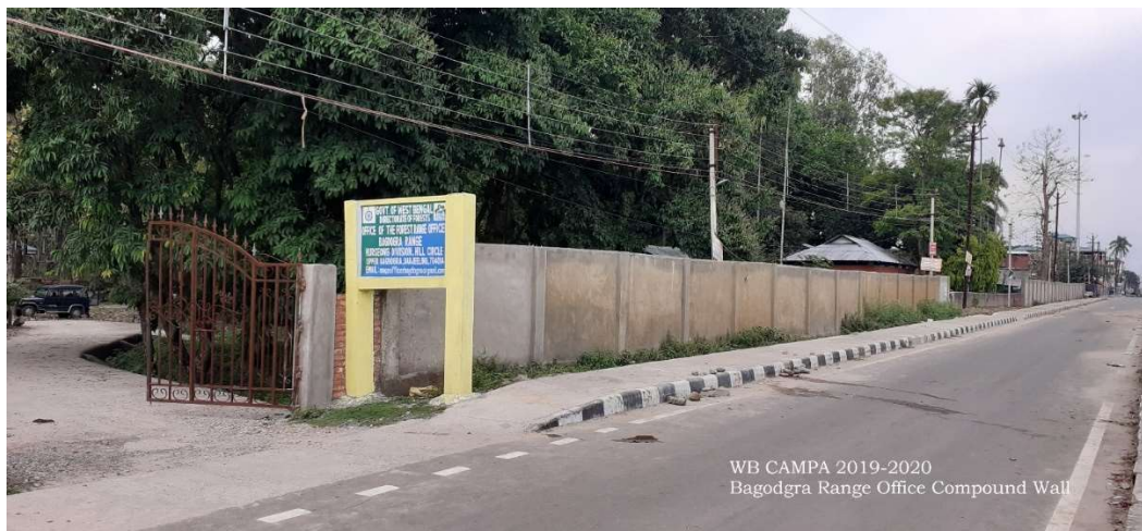
Office Compound Wall at Bagdogra Range in Kurseong Division 144 mts + 4.7 mts gate x 2 mts high above tie beam
